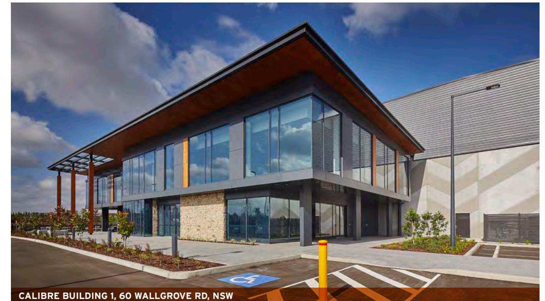
CALIBRE BUILDING 1, 60 WALLGROVE RD, NSW
