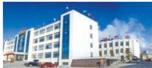
Yishui, Shandong Production Facility
