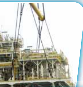
FPSO Stybarrow (Gas Treatment & Compressor Module)
