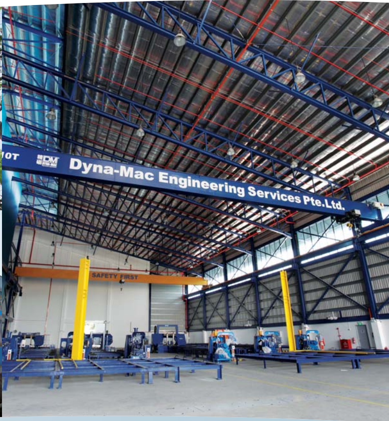
Constructed a new specialised pipe fabrication workshop at 13 Pandan Crescent
