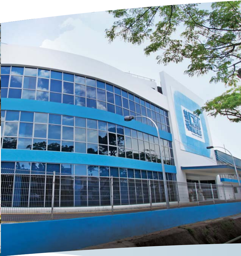
Launched a new 4-storey office building at 45 Gul Road
