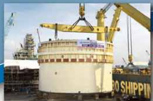
Bogie Support Structure
