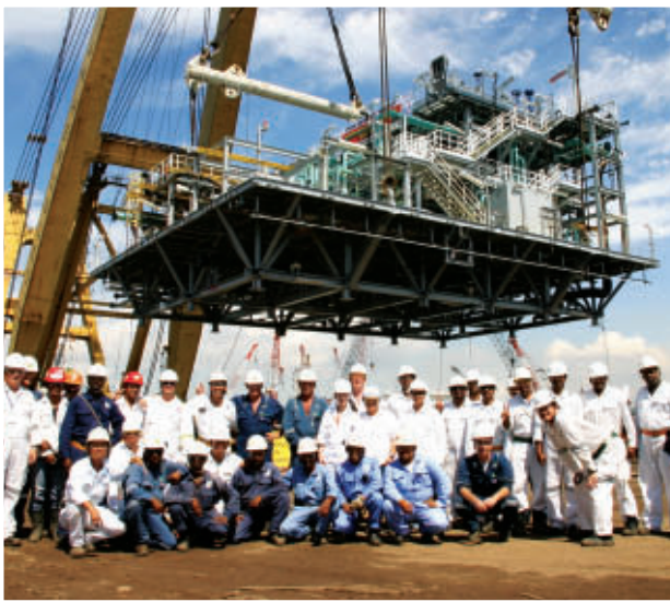
Last module load out for FPSO PSVM (VWS Westgarth), 12 August 2010
