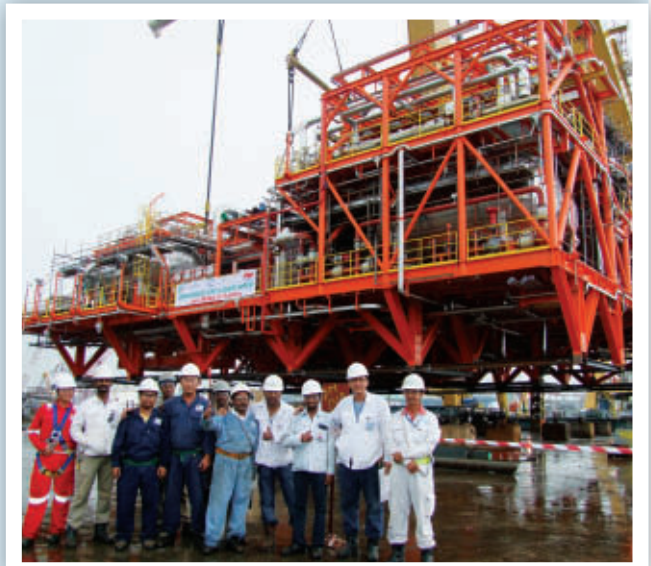
Last module load out for FPSO Armada TGT-1 (Armada TGT), 16 April 2011
