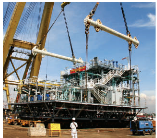
Last module load out for FPSO PSVM (Modec), 16 October 2010
