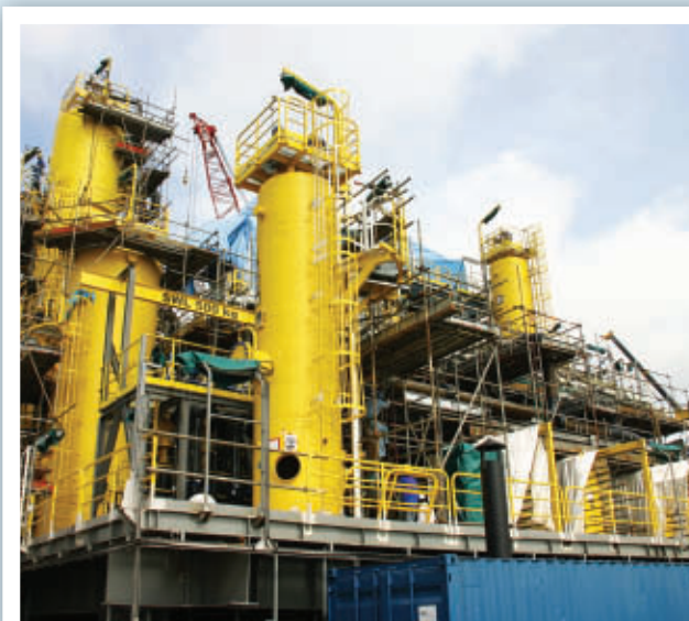
Last module load out for FPSO Aseng (SBM), 30 April 2011
