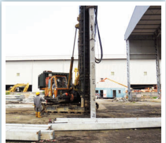
Commenced Construction of Specialised Pipe Fabrication Workshop, 15 May 2011
