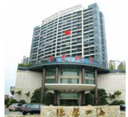
Our corporate office building at Jiangnan Mingju Phase 5
