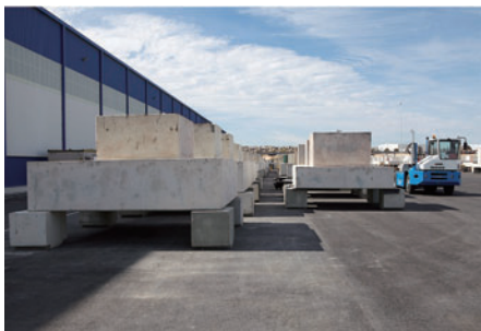
Pre-cast concrete foundations
