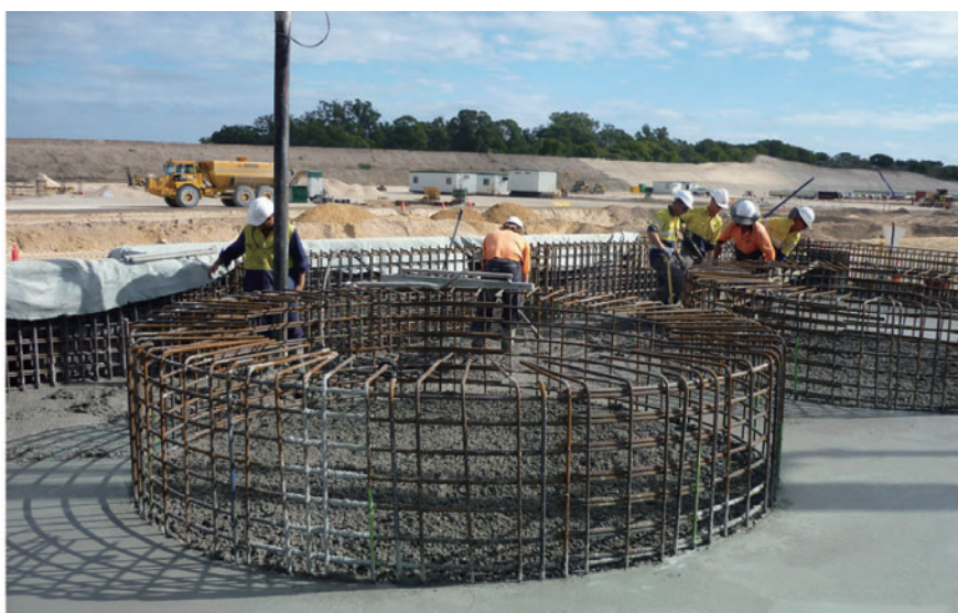
Site detailed earthworks and site concrete construction of steel work and equipment foundations, bund walls and slabs at the SSWA Binningup Desalination Plant
