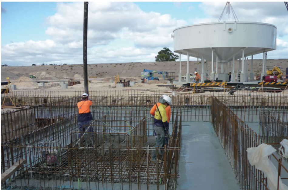
Detailed earthworks and concrete construction at the centrifuge transformer area of the SSWA Binningup Desalination Plant
