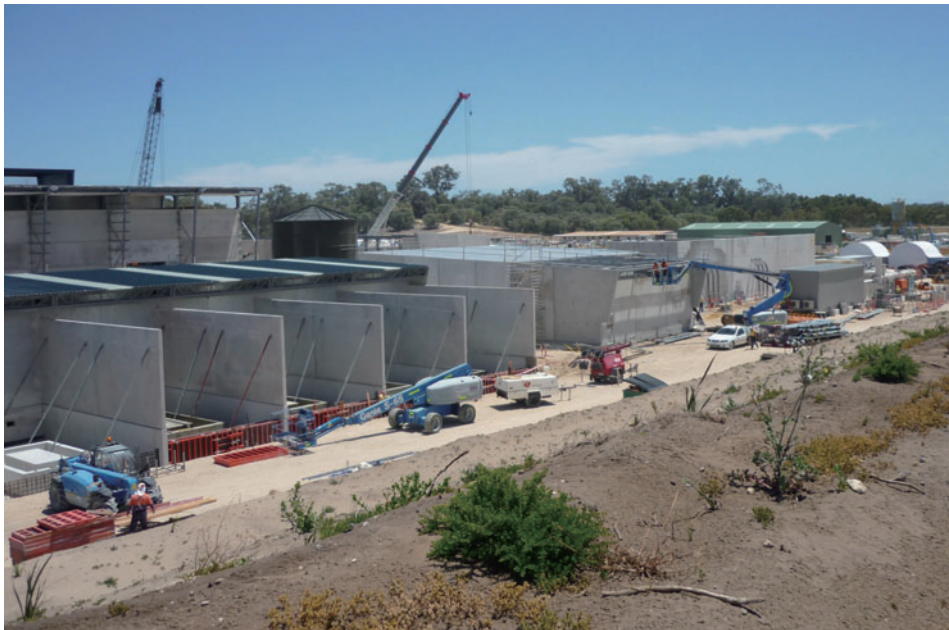
Detailed earthworks and concrete construction at the switch rooms of the SSWA Binningup Desalination Plant
