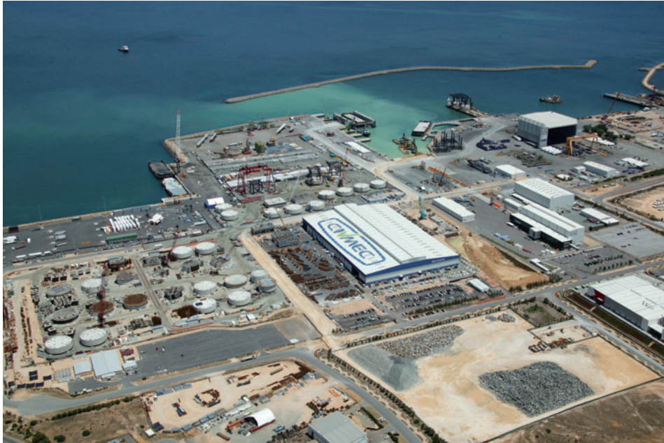
Aerial view of our Facilities
