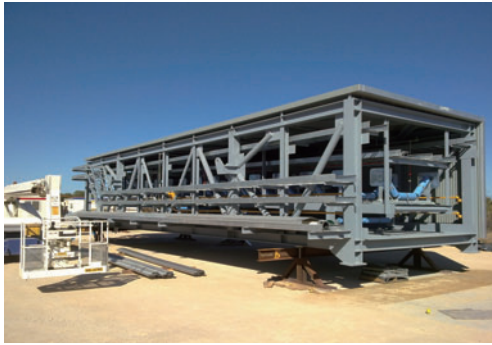
Fabricated modular assembly
