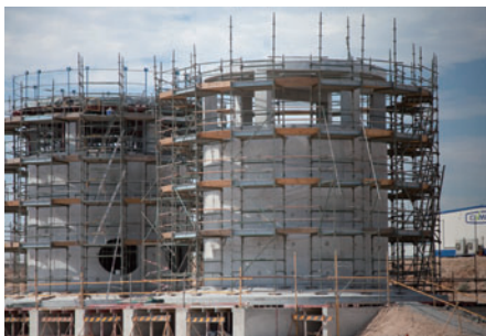
Pre-cast concrete seawater intake circular caissons
