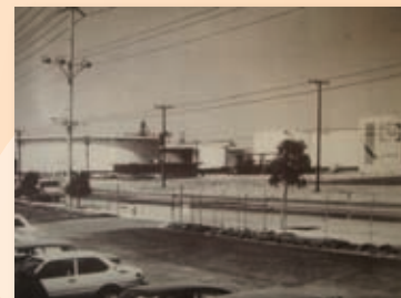
Chemoil's 1st storage terminal
