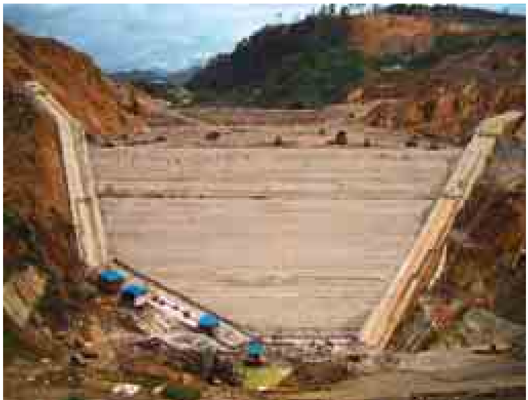
Top: View of the power tunnels at the Bakun Hydroelectric Project site
