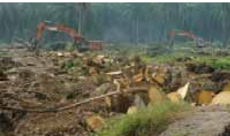
Zero-burning replanting technique is practised throughout Sime Darby Plantation's estates in Malaysia and Indonesia.
