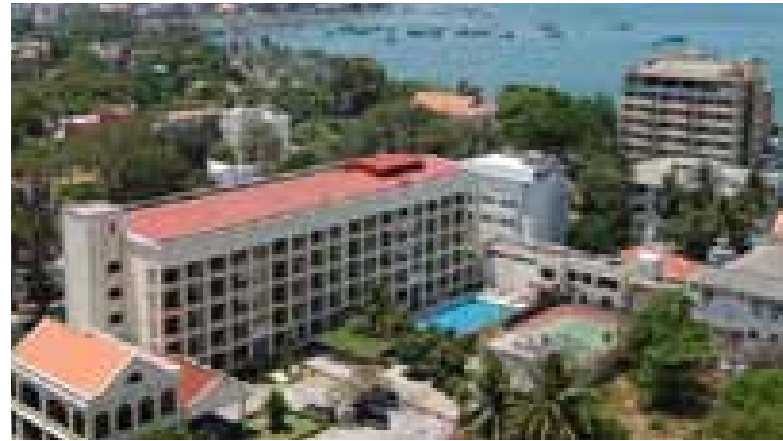
The Rangdong Orange Court in Vietnam
