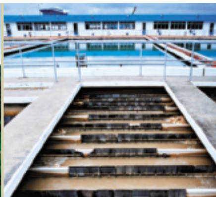
Flocculation chamber at Semenyih Water Treatment Plant
