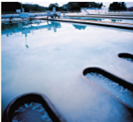
Settling tank at Semenyih Water Treatment Plant
