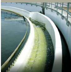
Inlet and Outlet of Clarifier for the Sewage Treatment Plant in Bayan Baru, Penang
