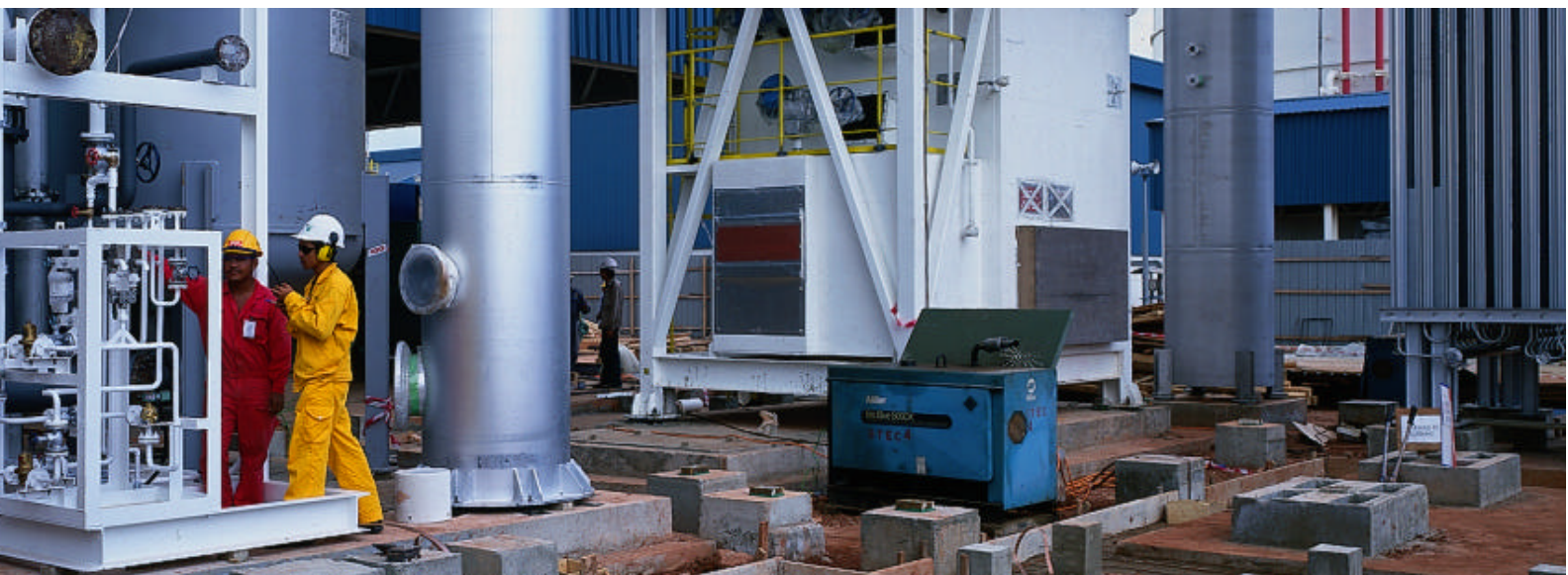
The construction activities of the additional unit of Nitrogen Generator Unit 2 (NGU2) at CUF Gebeng.
