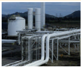
The ASU 1 plant which produces low pressure nitrogen and oxygen to the IPC customers
