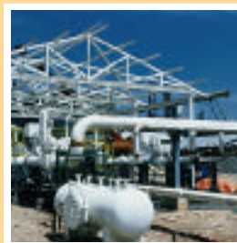
On-going installation works of ethane pipeline project in Kertih
