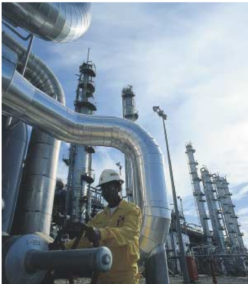
Left/Kiri : Plant Operator putting the heat exchanger in service Operator loji sedang mengaktifkan peranan penukar haba
