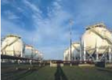
Top/Atas : LPG storage tanks Tangki simpanan Gas Petroliaam Cecair
