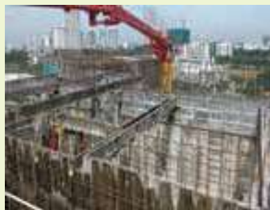
Aluminium formwork
