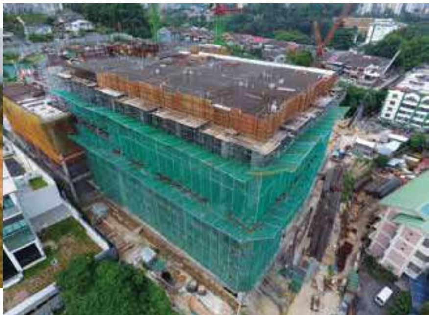
Work in progress at Residensi Gen, Kuala Lumpur
