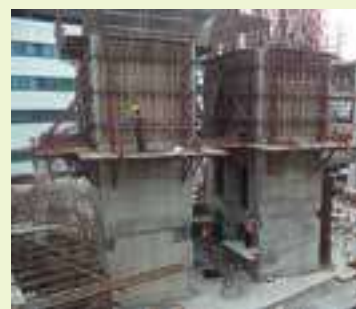
Normal Jump-form for lift core/ shaft
