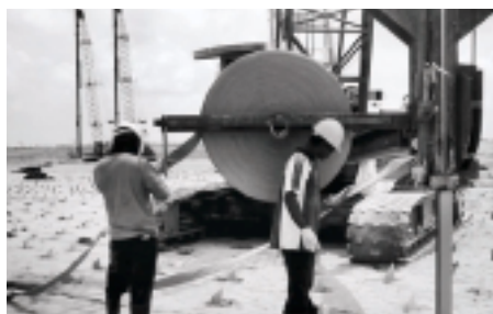
Reliance on Nylex for the supply of PVD earned Techniques Geosystems a world record for the fastest installation of PVD (Ground improvement works for Tanjung Bin Power Plant project).
