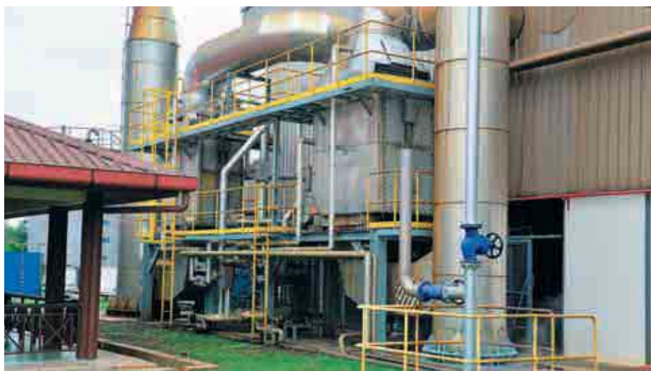
The Economiser is used to recover potential energy emitted from the boilers at our factories.
