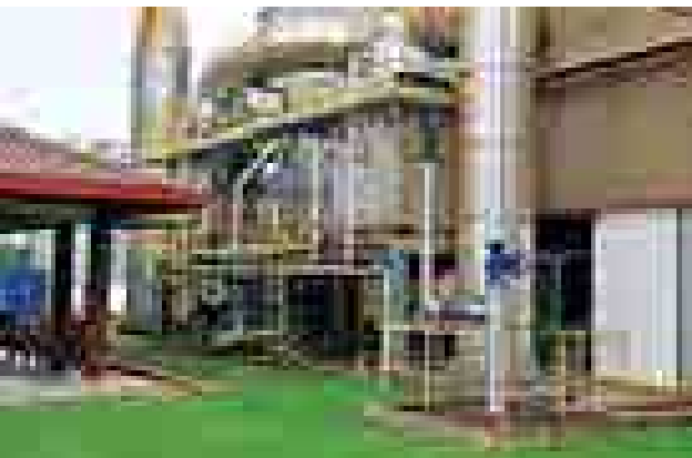
The Economiser is used to recover potential energy emitted from the boilers at our factories.
