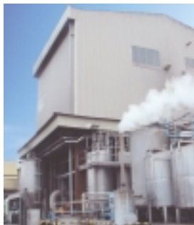
Coffee Waste Disposal Plant in Raja Muda Factory, Shah Alam Complex / Loji Pembuangan Sisa Kopi di Kilang Raja Muda, Kompleks Shah Alam
