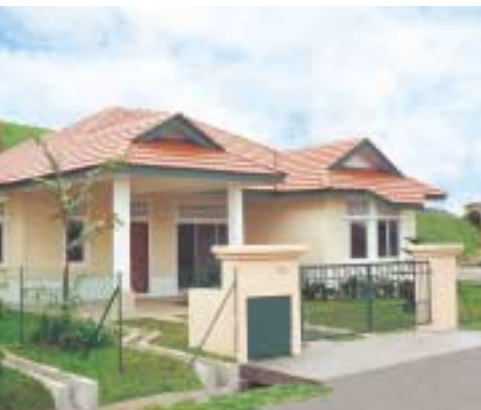
'Orchid' single-storey bungalow, Bandar Springhill
