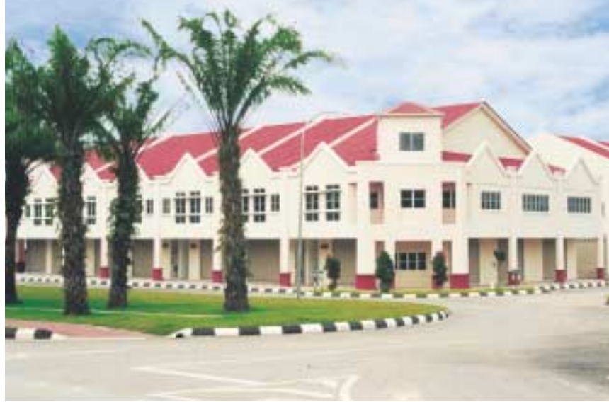
Newly completed double-storey shop offices, Bandar Springhill
