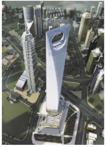
The Shanghai World Financial Center will be built by using Favelle Favco Tower Cranes
