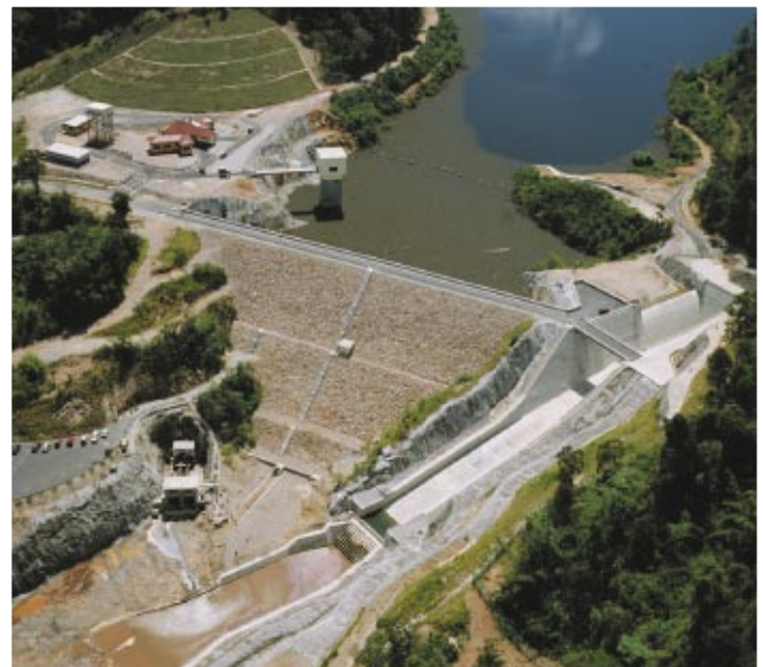
Beris Dam, Kedah built by Muhibbah Engineering (M) Bhd
