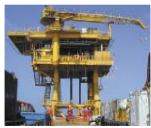
Favelle Favco Offshore Cranes on a project for Japan Vietnam, Petroleum Company Limited
