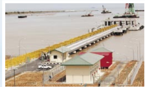
Palm Oil Terminal, Bintulu Port, Sarawak built by Muhibbah Engineering (M) Bhd
