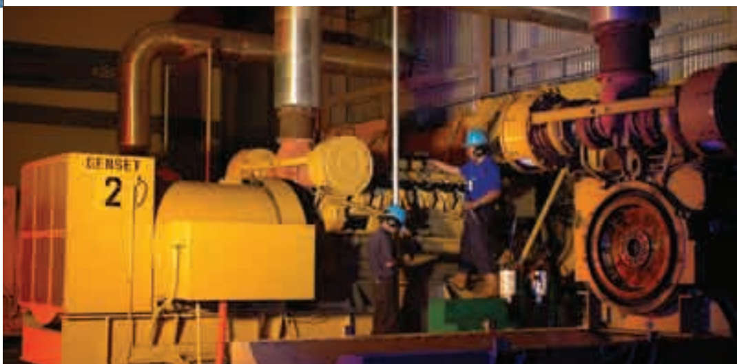
Genset major overhaul at PT Koba Tin, Indonesia.
