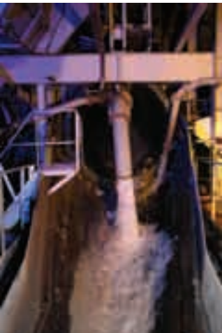
Revolving screen discharge.
