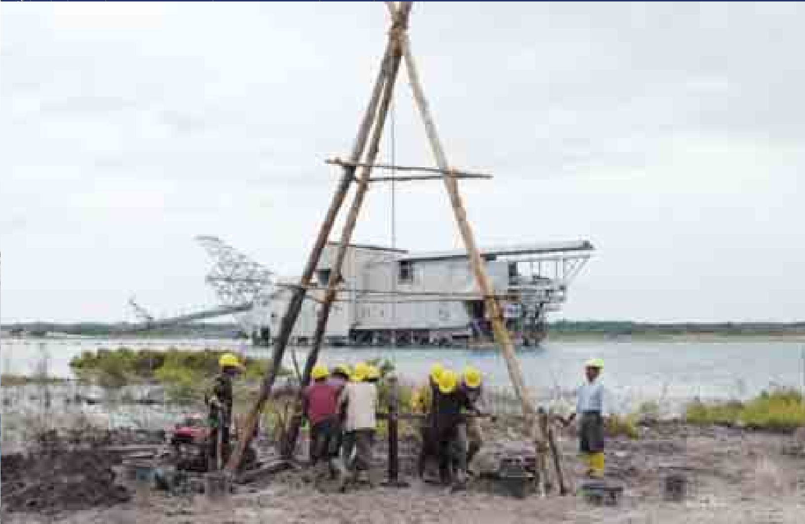
Check drilling ahead of Bemban dredge.
