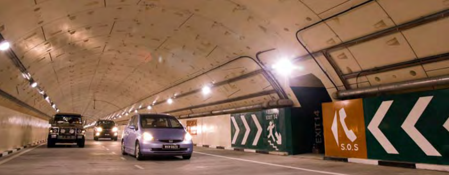
The SMART motorway, which forms part of the SMART flood bypass tunnel
