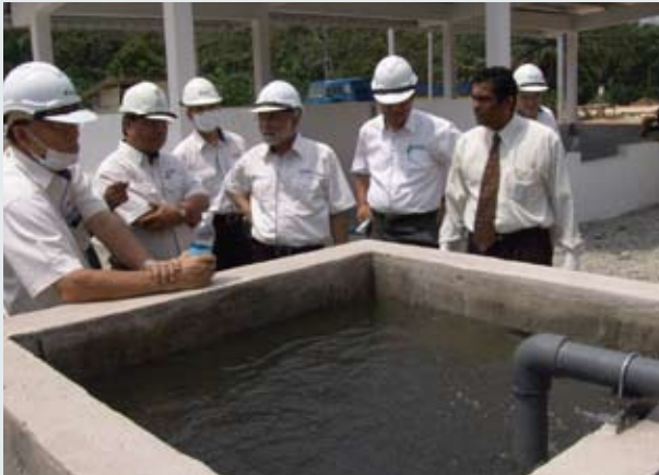
Board members visited the waste management and recycling centre of Recycle Energy on 15 March
