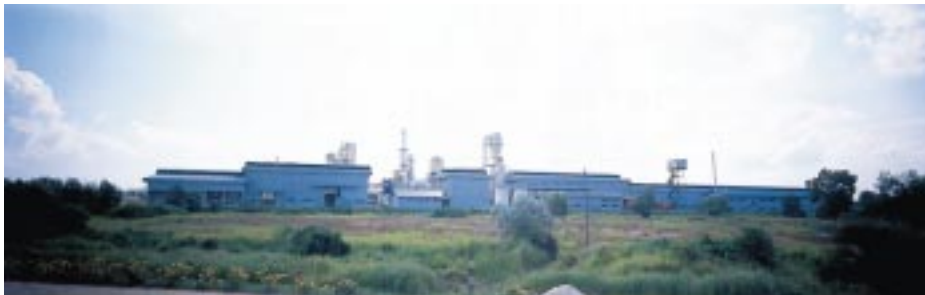
The chipboard plant at Gebeng, Kuantan
