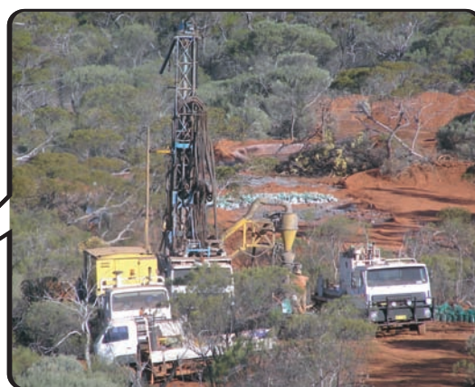
KARARA IRON ORE PROJECT SITE
