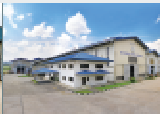
MYCRON STEEL FACTORY
