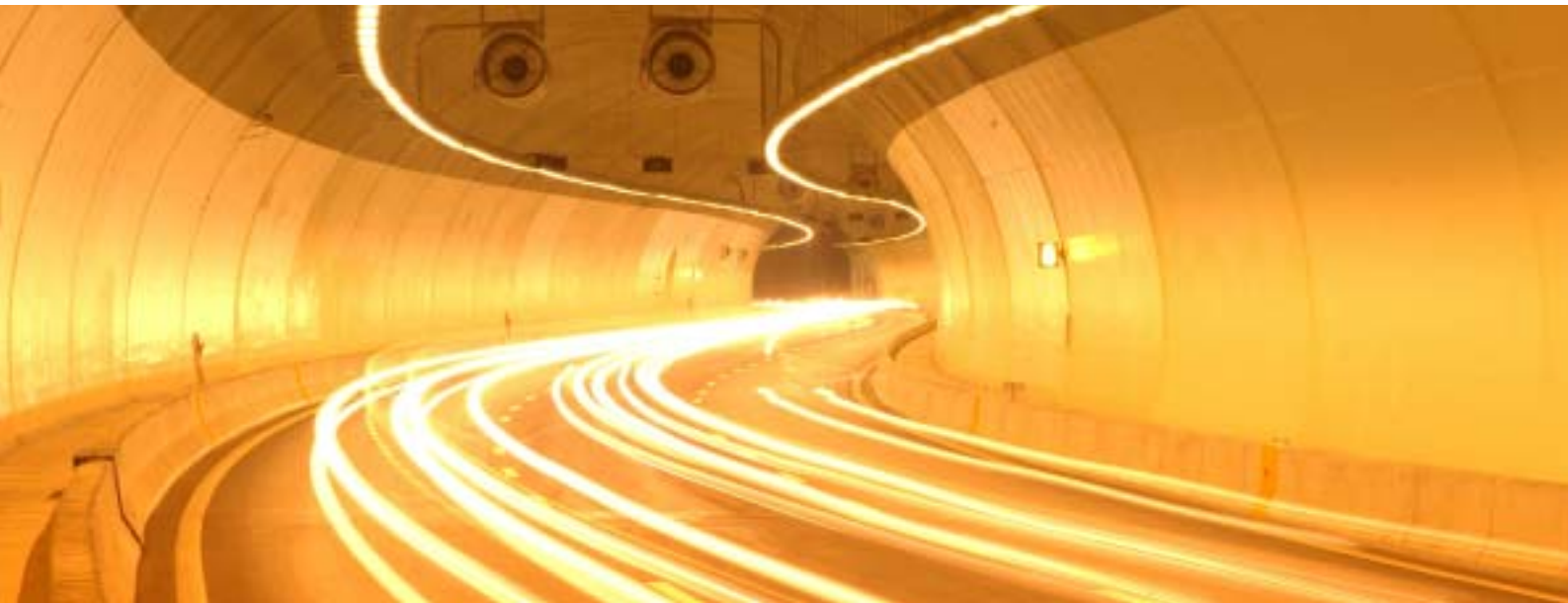
The state-of-the-art twin-bored Penchala tunnel
