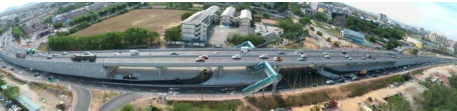
The substantially completed Kelana Jaya Interchange
