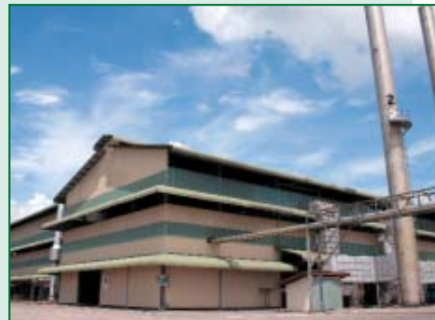
Kekayaan Palm Oil Mill, Johor – supermill of 120 tons FFB/hour
