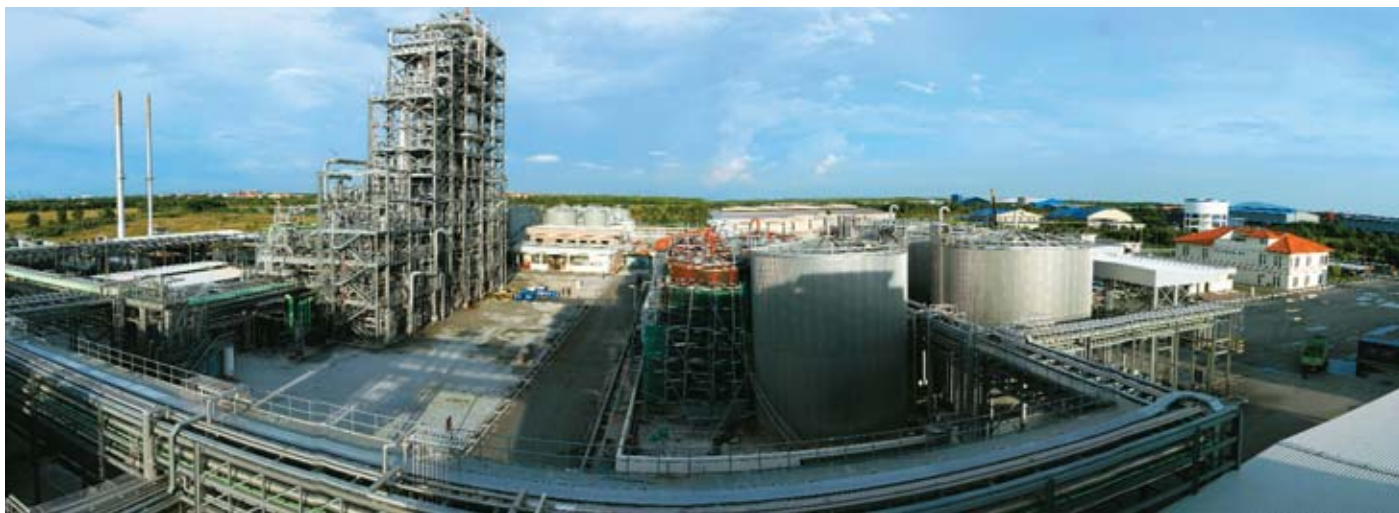
12.5 tonnes per hour Olemas fatty alcohol plant in West Port, Selangor, Malaysia
