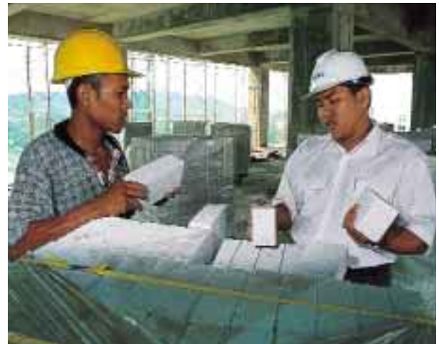
Work in progress at the Pejabat Kajicuaca in Petaling Jaya.
