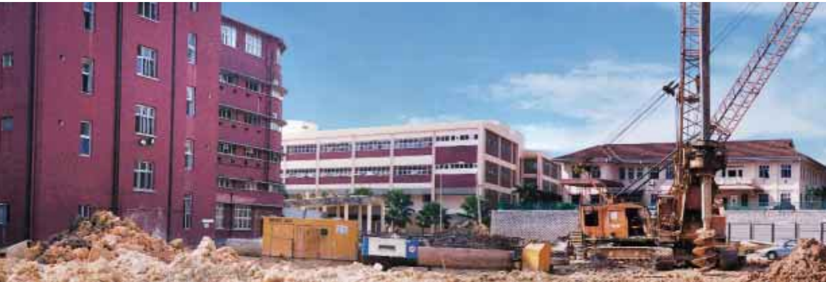
Extension works being carried out at Hospital Sultanah Aminah in Johor Bahru.
