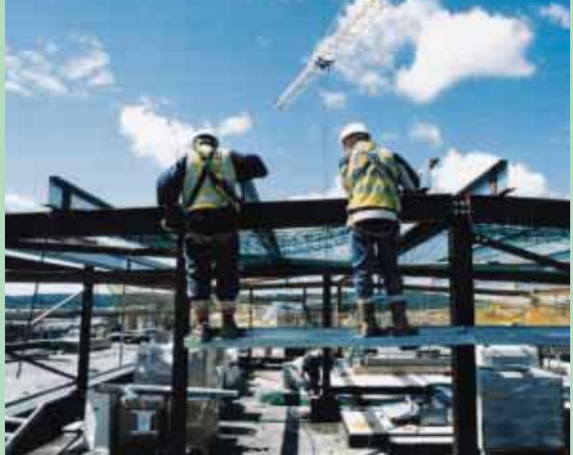
Construction works in progress at Bute Square.
