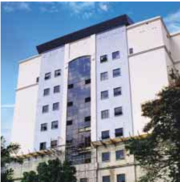
The extension works to the headquarters of the Pejabat Kajicuaca.
