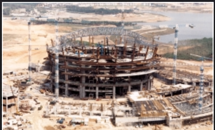
Construction work in progress at the Putrajaya Convention Centre (PCC). When completed, the PCC would consist of a circular Banquet Hall with a clear span of 75 metres, a Plenary Hall with 2,880 seating capacity, a Head of State Hall, Exhibition Halls and other state-of-the-art facilities.
