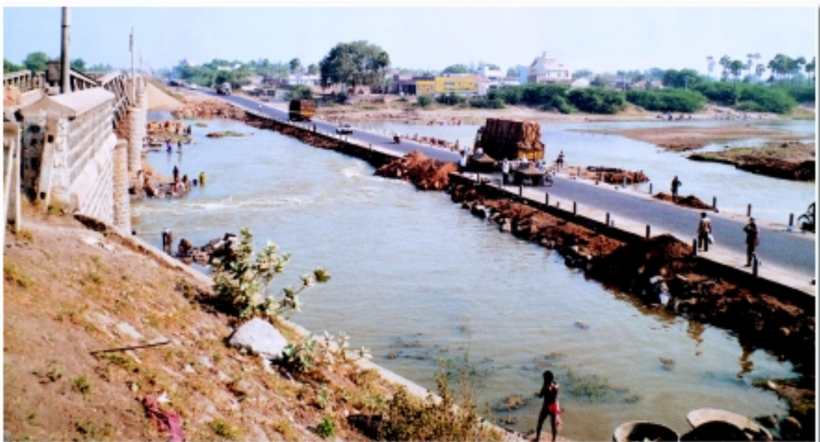
Chilakaluripet-Vijayawada Road Project, India: A temporary causeway / diversion constructed by IJM-Gayatri Joint Venture
