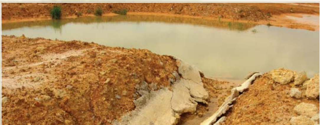
Silt trap built at the Bukit Cahaya Alam project in Shah Alam, Selangor
