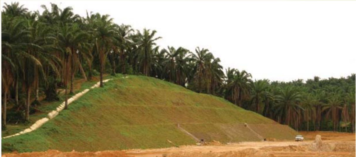
Turfing to prevent slope failure
