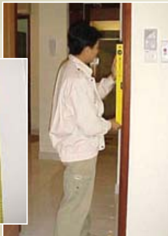
Checking of door frame alignment
