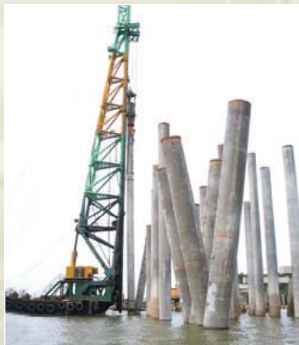
Installation of the Ø1200 mm ICP piles at the Independent Oil Terminal, Kg. Senai Port, Sarawak
