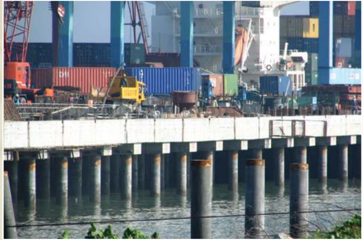
ICP Piles - supporting the wharf of West Port in Port Klang, Selangor
