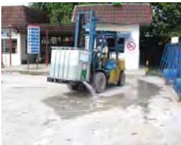
Forklift carrying water tanks are used to water the roads to contain dust
