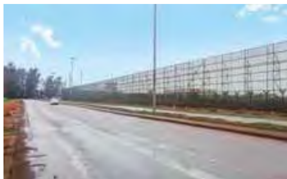
Airborne dust mitigation panels at Kuantan Port
