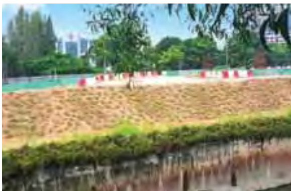
Spot turfing as slope protection
