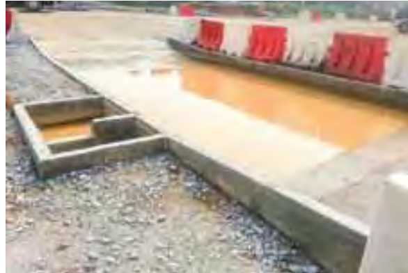
Wheel washing facility provided at site entrance
