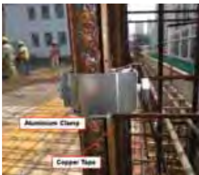
Provision of aluminium clamp for fixing of copper tape for earthing purpose
