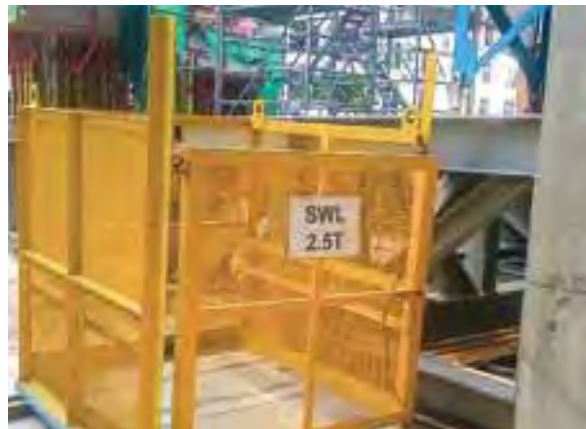
Material lifting cage for safe lifting operations at site
