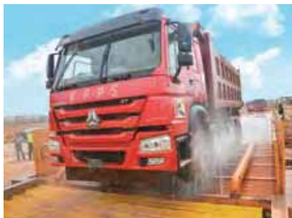
Wheel washing facility to minimise dust pollution
