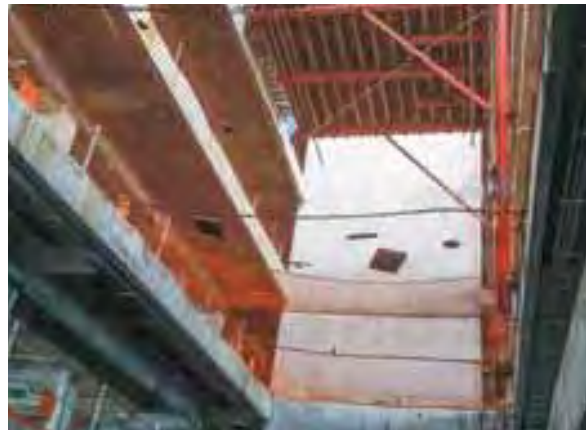
Safety nets are used to prevent falling hazard
