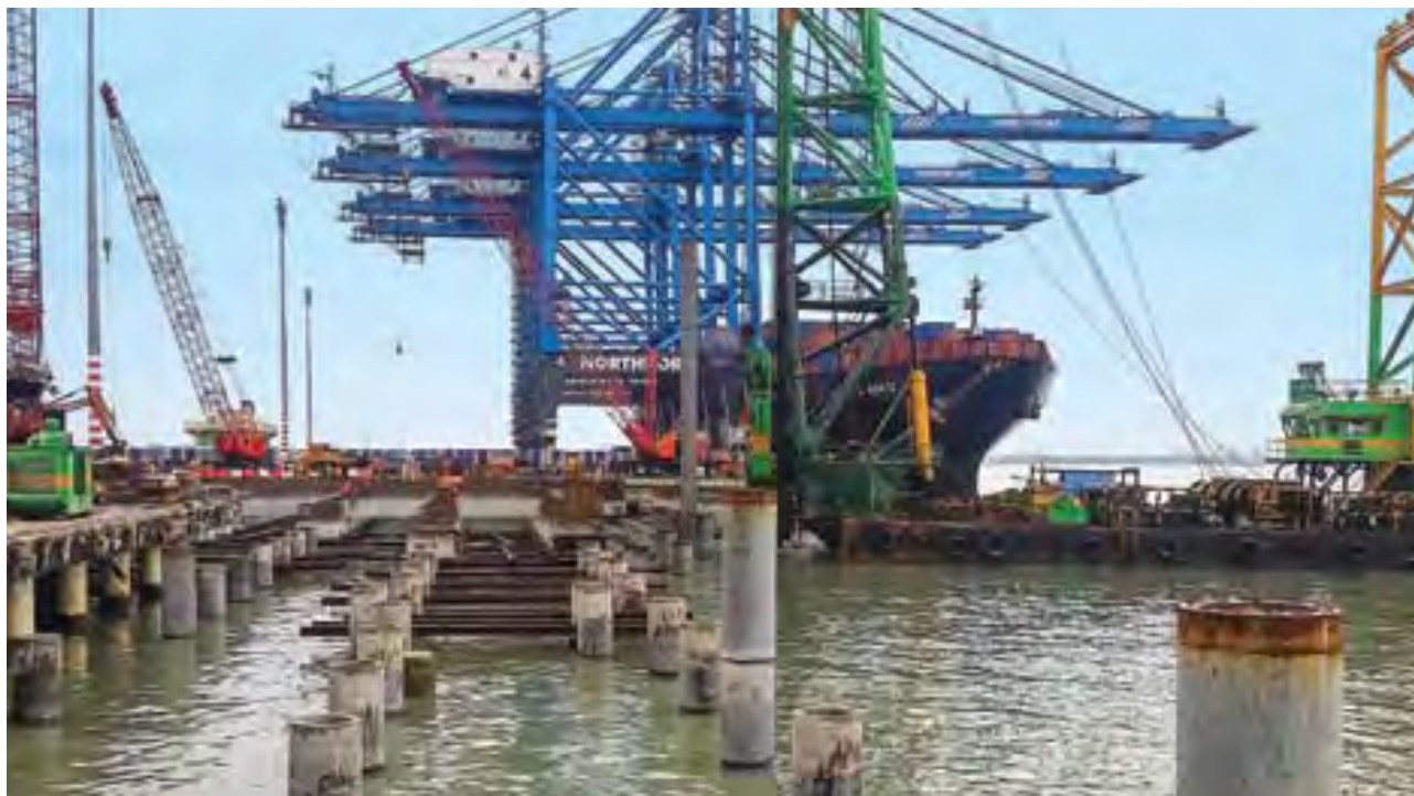
ICP Piles used at Upgrading works of North Port CT4, Wharf 8, Port Klang
