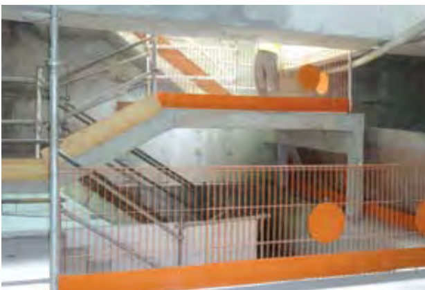
Installation of fencing to prevent falling hazard
