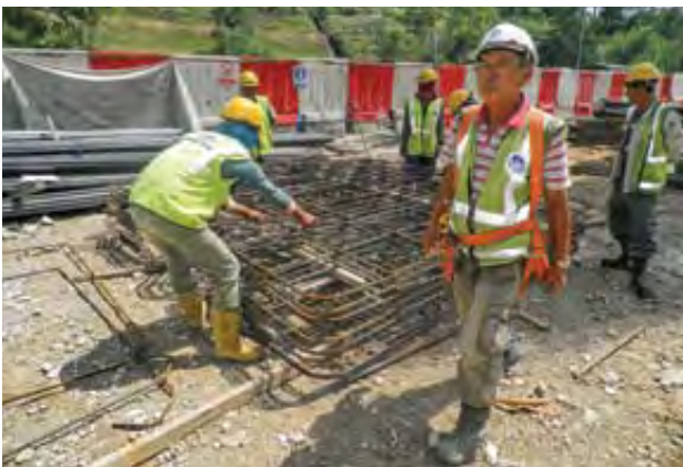
Standing supervision by supervisor is adhered to ensure proper protection and care while fabricating reinforcement at the Cheras Sentral Section, MRT V5 Project
