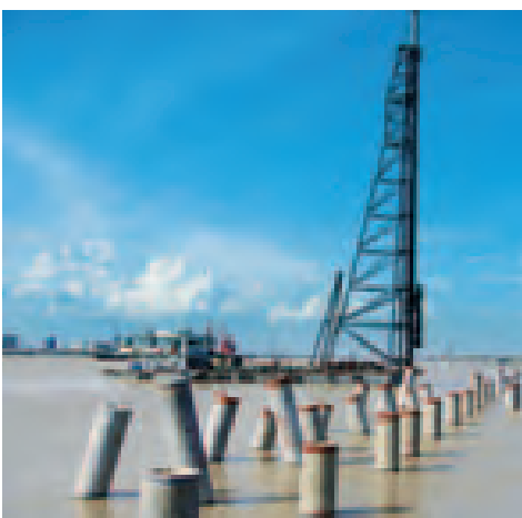
Piles at the Haiwan Petrochemical Port, Dongguan, China
