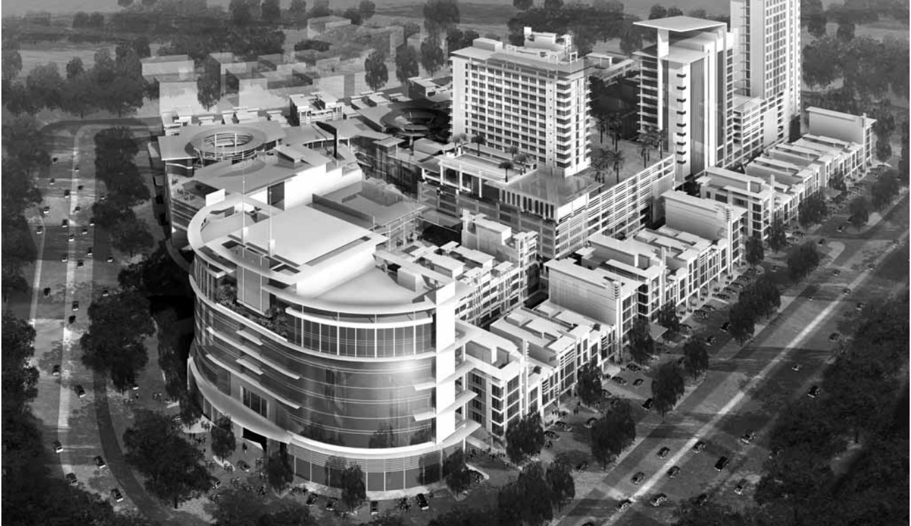
Phase 1 covers 20 acres on the eastern side comprising shop offices, corporate offices, retail suites and Citywalk
