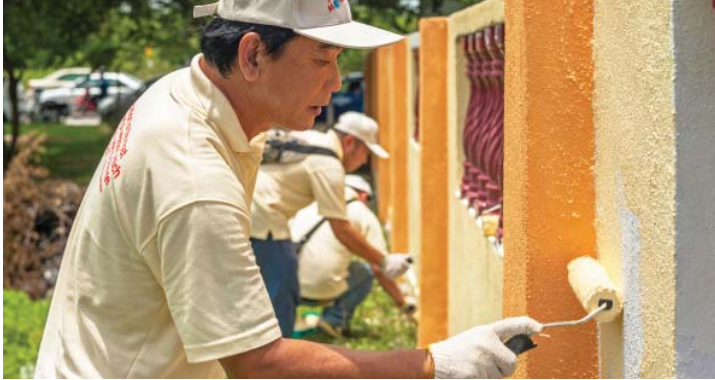
Employees repainting premises of a school during the Big Day Out 2014.
