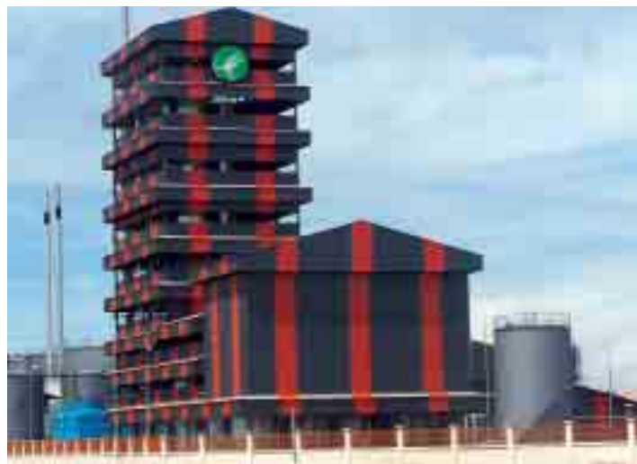
Austral Edible Oil refinery in Bintulu, Sarawak a new addition to the Division's refining facilities.
