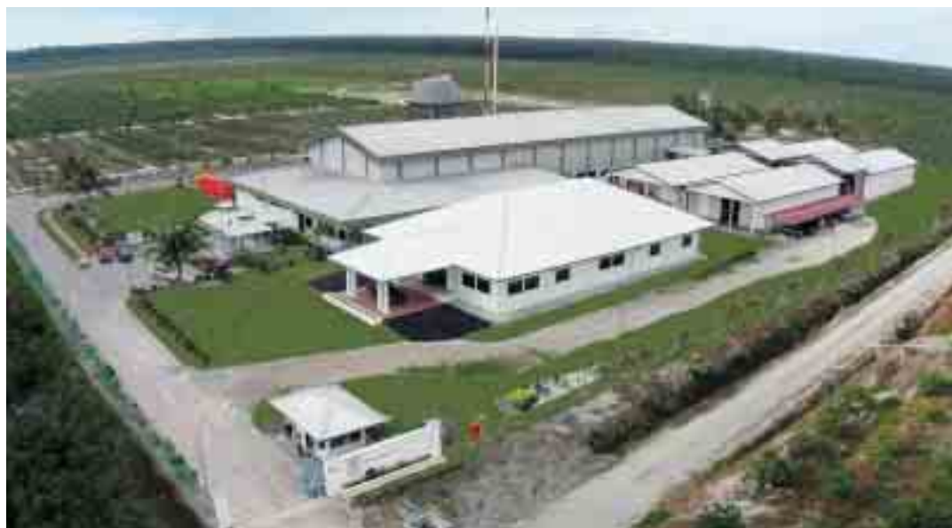
Centrifugal Process Sdn. Bhd.'s new factory and administration building within the Sg. Wangi pink guava plantation.
