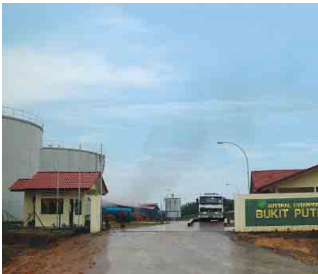
Bukit Puteri Oil Mill is the new addition to Golden Hope's stable. The mill will be equipped with continuous steriliser.
