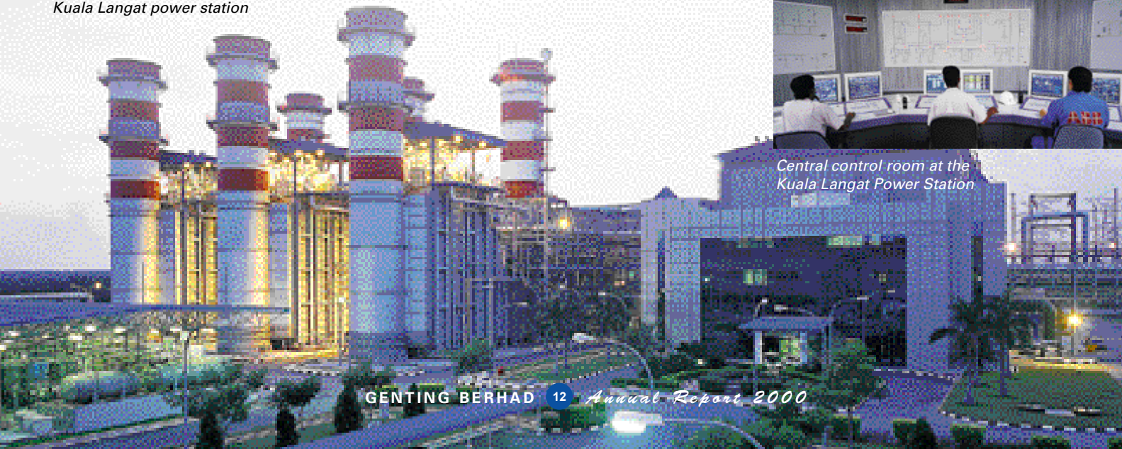
Heat recovery steam generators at Kuala Langat power station
