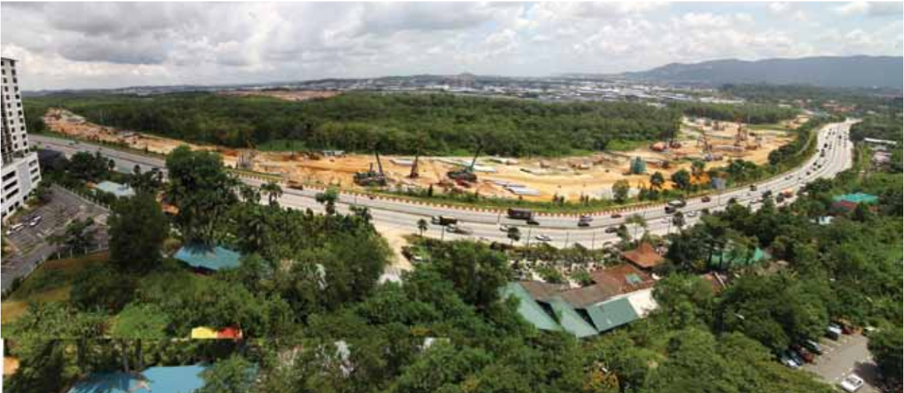
Progress of Klang Valley My Rapid Transit (KVMRT) Project
