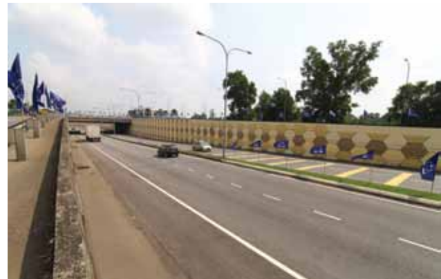
Completed Senawang Interchange
