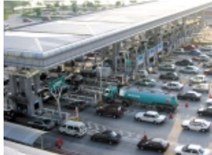
left: The LDP toll plaza at Bandar Sunway.
